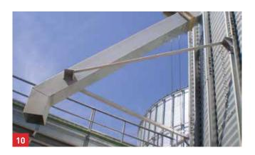
For capacities up to 600 t/h, the catwalks are modular with open type frames, while for high capacity and heavy-duty conveyor systems, they are modular and lattice framed.
